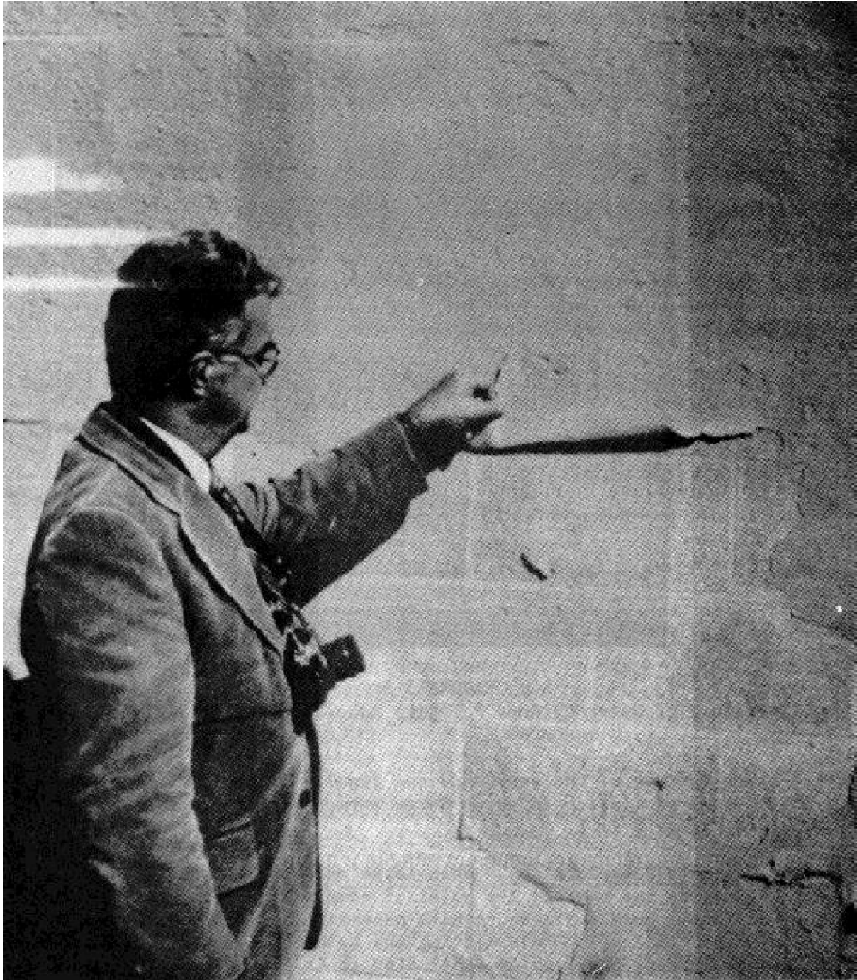
FIGURE 5-4 Failure of Solvent-Thinned Paint To Adhere to Chalky Surface
