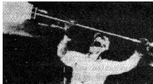
FIGURE 4-13 Flame Cleaning
